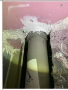
In the service risers within each of the blocks, at top floor level, plastic pipes appeared to pass through the ceiling into the void above and it could not be confirmed whether suitable wraps or similar were used to prevent possible fire spread. No intumescent collars or intumescent fire stopping materials were observed. In the event of a fire where inadequate fire stopping materials are used a fire may be able to spread from a service shaft, placing persons at risk of harm.
