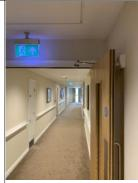
Electromagnetic corridor doors held open on auto door release devices are not released at night, to allow the free movement of the residents, but the doors are routinely tested and are linked to the fire alarm system. Detectors were seen to be in place in close proximity to the doors on the corridors.
