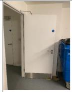
The inner lobby door to the refuse room in Block B was wedged open at the time of the assessment. Refuse rooms are considered to be higher risk rooms and the 2 x 30 minute fire doors in place are required to maintain the 60 minutes fire separation between the corridor and the refuse room itself. Where this standard of fire separation is not maintained, persons may be placed at risk of harm.
