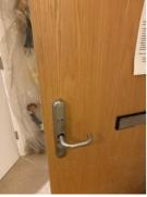
On the internal side of the flats accessed, lever handles were observed which ensure that persons do not require the use of a key to exit their flat.
