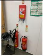
CO2 and wet chemical firefighting equipment is provided in the kitchen of the Hub, as is a fire blanket.
