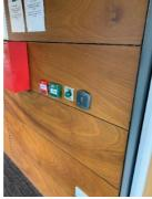
Certain final exit doors are provided with a sliding power assisted opening mechanism. Assurance was provided that these are linked to the fire alarm and open upon its activation. A 'Green Box' emergency override is also installed adjacent to the doors and opens the doors when activated.
