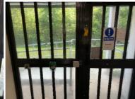
8.21 The emergency override on the escape side of the electromagnetically secured laundry door is not labelled as an override.
