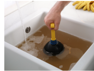
Clearing blocked sinks, basins, and showers
