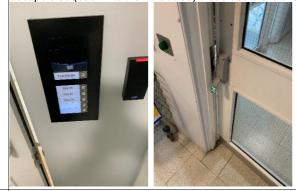
8.18-8.19 Where electromagnetically secured doors are installed within the premises (e.g. final exits, external exit from the forecourt, laundry), these were observed to be accompanied by suitable green box emergency overrides. However, see the above finding
