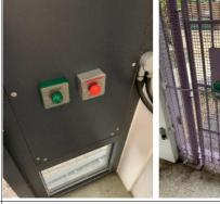
8.18-8.19 As part of WCHG's standard responses, they have confirmed that due to most FRAs raising a finding, WCHG had engaged with Tech Sol and confirmed that doors fail safe/open upon a fire alarm activation or loss of electricity, and that break glass points are installed as a back up should the push to exit button fail.
