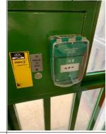
8.21 The previous FRA raised an action in relation to the escape side of the electromagnetically secured laundry door, both release devices are identical, these being 'push button to exit' devices, and neither of the buttons was labelled as the override. The previous FRA action has been signed off as complete on 27/07/2023. Onsite observations showed that one of the buttons is now labelled as previously recommended.
