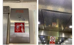
12.14 Although the common fire alarm system is not a purpose-designed Evacuation Alert System (EAS), the previous assessor was informed that it had been re-configured so that the Fire and Rescue Service could sound the fire alarm system on a chosen fire floor and the floors above and below the chosen floors, initiating evacuation.
